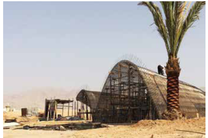
Completed Ayla Golf Comfort Station structural framework Photo credit: Oppenheim Architecture
